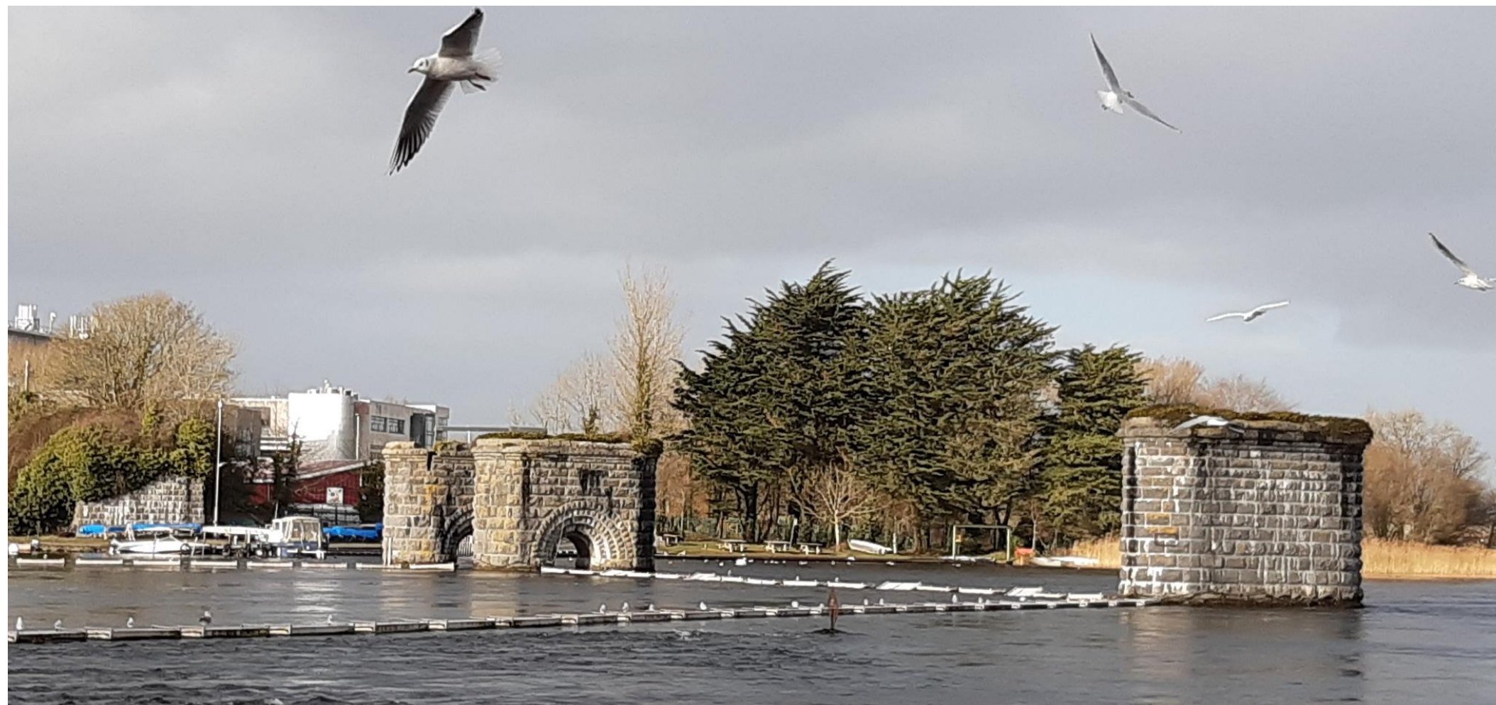
Existing piers which used to support the Clifden Railway Bridge
